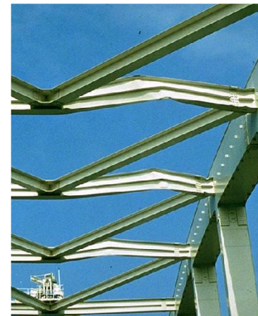
Riostras de acero, Kobe, 1995 (Annotated Slide Collection, EERI)
