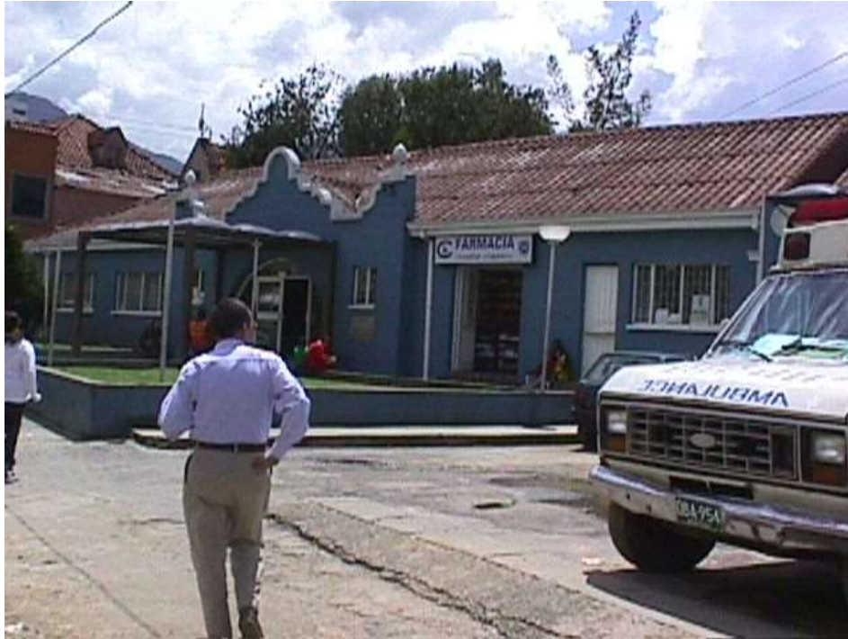
FACHADA PRINCIPAL HOSPITAL DE CHAPINERO
